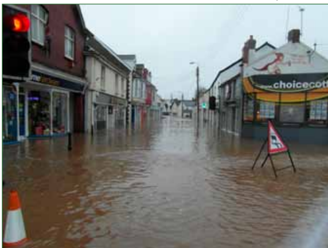
Flood gap: the new scheme will need to cover businesses too
